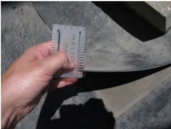
Figure 6: 90 mil membrane thickness at lower roof section
