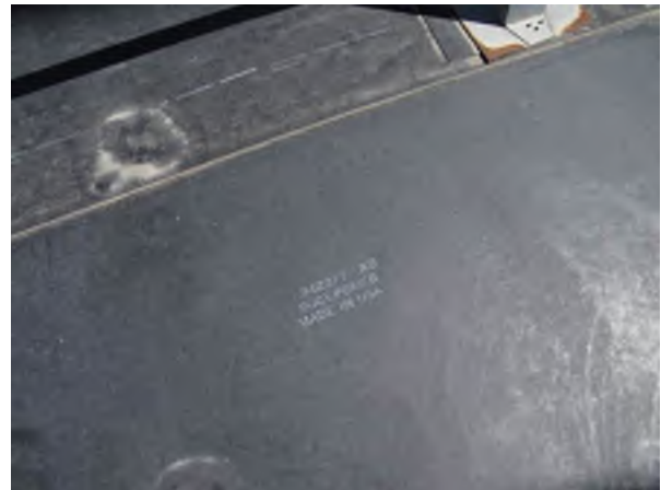
Figure 7: Label indicating 60 mil membrane thickness at upper roof section
