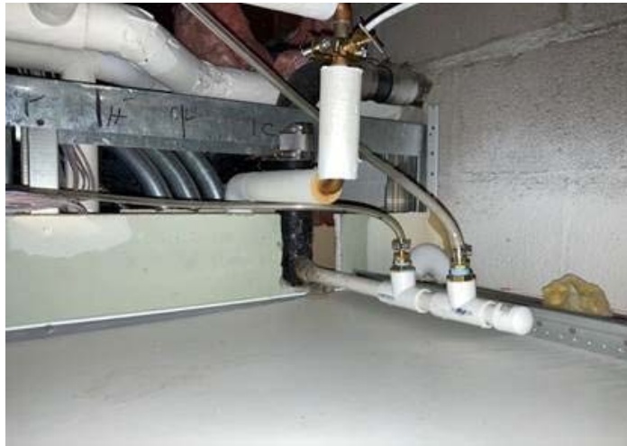
Basement Plenum Ceiling
